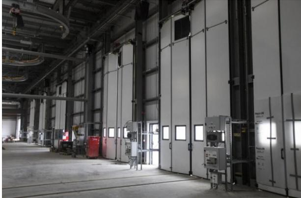
The doors are operated by a powerful, centrally mounted SEW drive unit, combined with a purpose designed control panel incorporating inverter control for smooth starts and stops. The system takes less than eight seconds to full open and close, and safety is ensured with full height pressure sensitive safety edges and photocell beams to create a safe zone
