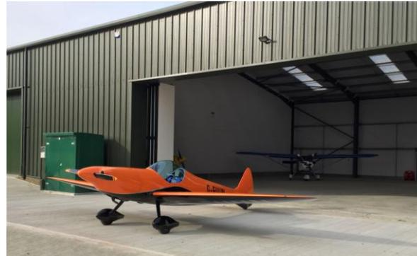
The new building is 110 m wide x 24 m deep and comprises two 1150 m<sup>2</sup> hangars which will each accommodate between 12 and 18 aircraft. Between the two hangars is a 290 m<sup>2</sup> fire station which will house one large fire appliance and 4 smaller Land Rover appliances.
