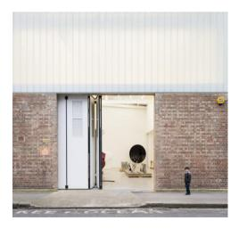
Jewers supplied manually operated Osprey sliding, folding doors in four and five leaf configurations. Manufactured as a single piece construction, each of the door panels is fully insulated with environmentally friendly insulation materials which optimise thermal efficiency and reduce noise pollution by up to 25dB. The doors incorporate soft compound weather seals to all edges, which also protect against finger and toe trapping. Some of the doors are fitted with louvres to
