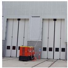
insulated, single piece steel faced composite panels operated by a powerful, centrally mounted SEW drive unit. Control is via a purpose-built PLC control panel incorporating remote status reporting and inverter control for ultra-smooth operation.
