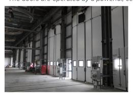
purpose designed control incorporating inverter control for smooth start and stop and takes less than eight seconds to open fully. Safety is ensured with full height pressure sensitive safety edges and photocell beams to create a safe zone around the door during operation. An electro mechanical lock within the motor automatically holds the door in the closed position while automatic solenoid floor bolts provide additional security and protect against high winds.
