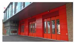
stations where appliances need to exit rapidly under 'blue light' emergency response conditions. That's less than half the time it takes for typical vertical lifting doors to open. In the event of power failure, each door can be instantly and effortlessly opened by hand in under 10 seconds.
