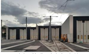
servicing at any one time. MDS were commissioned by the principal project team of Coleman Rail and Architectus to supply and install automatic bi-folding doors which are fitted to the six LRV entrance roads into the Lilyfield depot.
