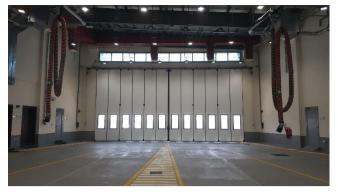
double glazed vision panel, and is fitted with multi-wall rubber seals to all edges to reduce water, air and dust ingress.
