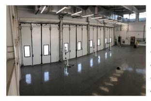
Each door is 4.3m wide x 4.3m high and is configured in four leaves with two leaves folding neatly to each side of the opening. 600mm x 1200mm double glazed toughened glass windows set in thermally broken aluminium frames are fitted in each door to improve driver vision and interior illumination. Swift doors are
