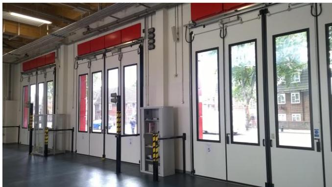
around the door which greatly reduces the risk of an impact ever occurring. In the event of power failure, each door can be instantly and effortlessly opened by hand in around 2 seconds.
