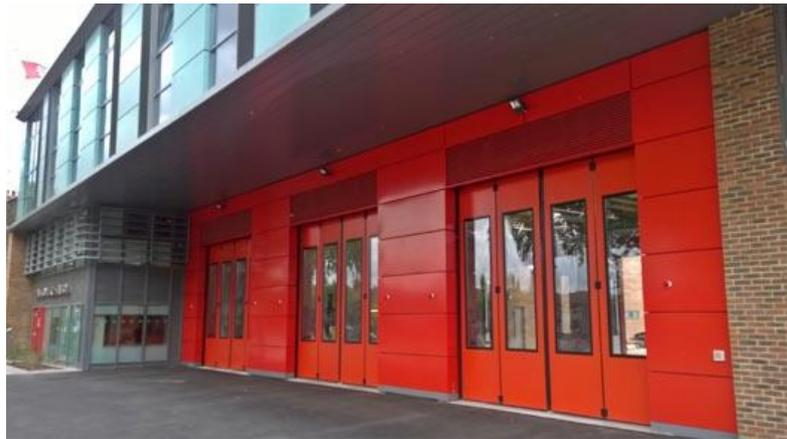
Doors. “The Swift door opens fully in less than 7 seconds, making them ideal for fire stations where appliances need to exit rapidly under ‘blue light’ emergency response conditions. That’s less than half the time it takes for typical vertical lifting doors to open.”
