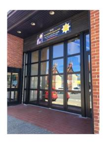
Jewers constructed the new doors using durable galvanized steel frames which were finished with a black powder coating. The doors were glazed to full height using 24mm thick low-E, argon filled double glazed units to allow good visibility and natural lighting whilst maximising thermal efficiency. This not only ensured they matched the appearance of the earlier doors, but would have a long life and require minimal maintenance.
