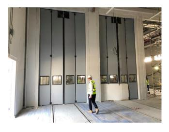
Doors are operated by a powerful, centrally mounted SEW drive unit, combined with a purpose designed PLC control panel incorporating inverter control for smooth operation. Opening time is under eight seconds, and in the event of power failure, a low-level disengage handle enables the doors to be instantly opened from ground level.
