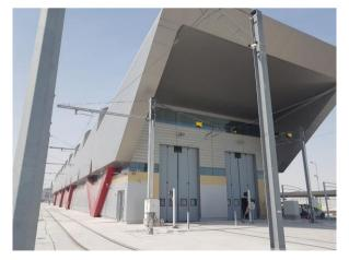
The thirty sets of 6.45m high electrically operated Swift-SEW doors were installed on three depot buildings. Six sets are on the Service Station, which incorporates the wash bay, twelve sets within the Maintenance Building and a further twelve sets on the Stabling Depot, which houses the trams when they are not on the dusty streets of Qatar.
