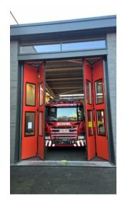
alarm is activated. This ensures that the doors are fully open when the fire tender is ready to depart. In the event of power failure, it takes only 2 seconds for each door half to effortlessly be opened manually.
