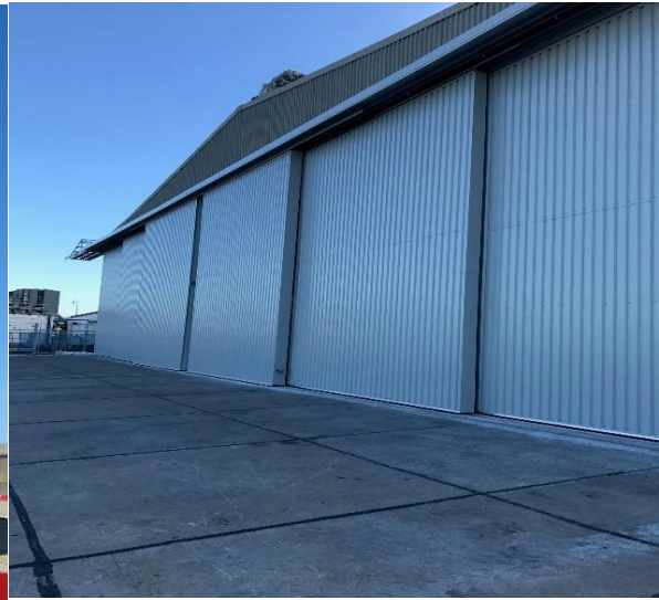
T2 Hangar – New Esavian Type 126 Doors
