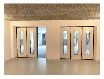
Doors are configured in 3 leaves fitted within a made to measure cold-rolled steel frame with a built-in threshold plate and a discreet top track. The odd leaf is used as a pass door when the full opening is not required and is fitted with a pair of lever handles and two deadlocks for additional security. Each leaf is fitted with a 300mm wide by 1500mm high double-glazed window to allow plenty of
