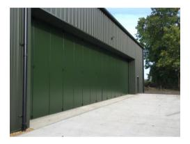
into the bottom and top track. A lever handle withdraws each bolt to allow the door leaves to be easily pushed aside to create the wide openings.
