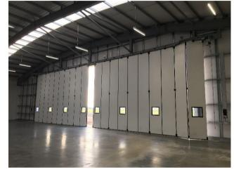
powerful inverter controlled drive unit which moves each of the 10 leaves effortless across the opening and then folds them into a 1m<sup>2</sup> footprint behind the opening.
