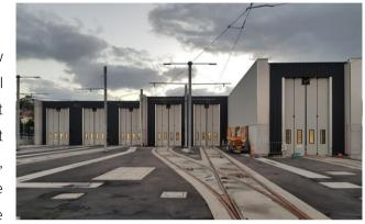
than 9.7 million customers each year. The Lilyfield Light Rail maintenance depot building, along with a 2<sup>nd</sup> depot at Randwick will house the facilities needed to service and maintain the light rail vehicles (LRVs) and Lilyfield can accommodate up to six LRVs for servicing at any one time.
