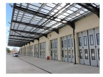
automatically. In the event of power failure, each door can be instantly and effortlessly opened manually via low-level disengage handles to prevent delays.
